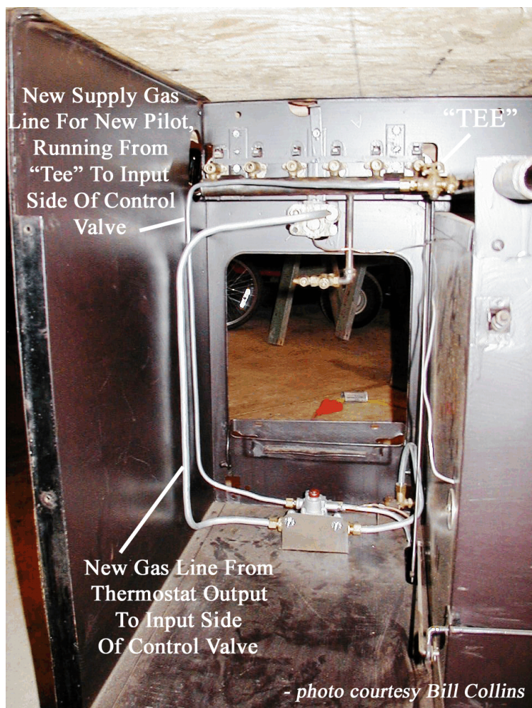
Figure 7 - New Gas Lines From Thermostat & From "Tee" To To Control Valve Installed.
